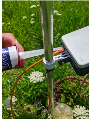
Applying silicone to PoE plug to stop moisture
